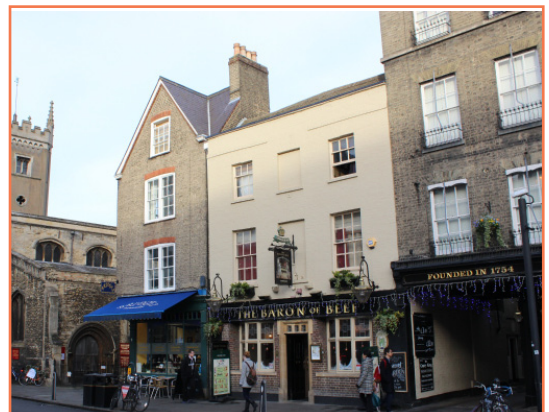
Three storey buildings at Bridge Street junction
