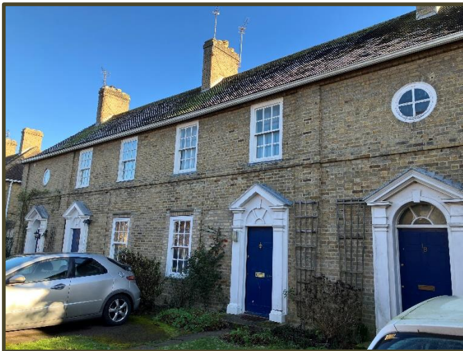
Above: Nos. 1A, 1B, 2A and 2B showing building details
