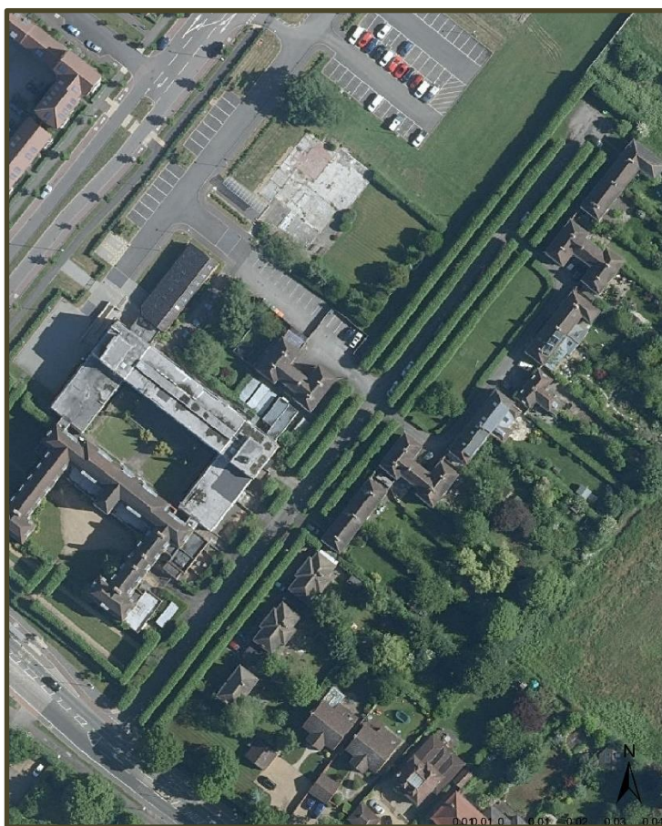
Above: 2018 Aerial view of Howes Place and the former NIAB Headquarters Building
