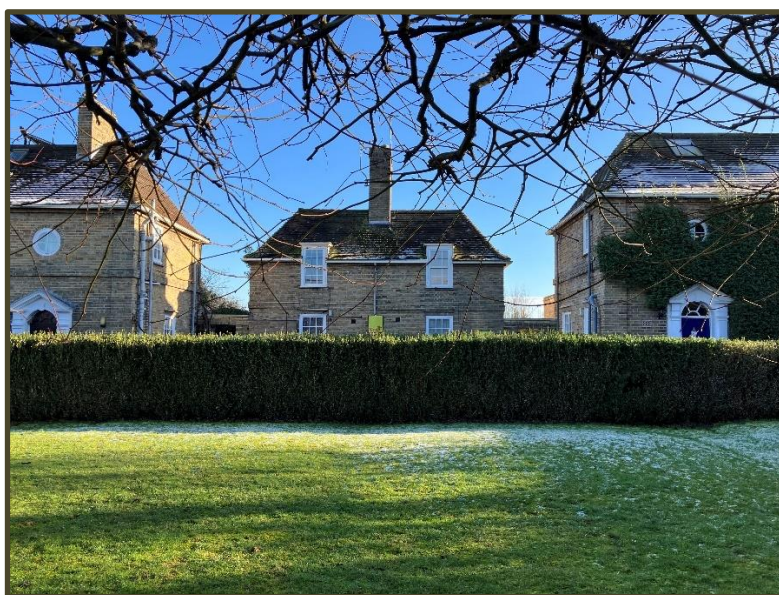
Above: Nos. 6A and 6B Howes Place, the former boiler laundry room, overlooking the central green
