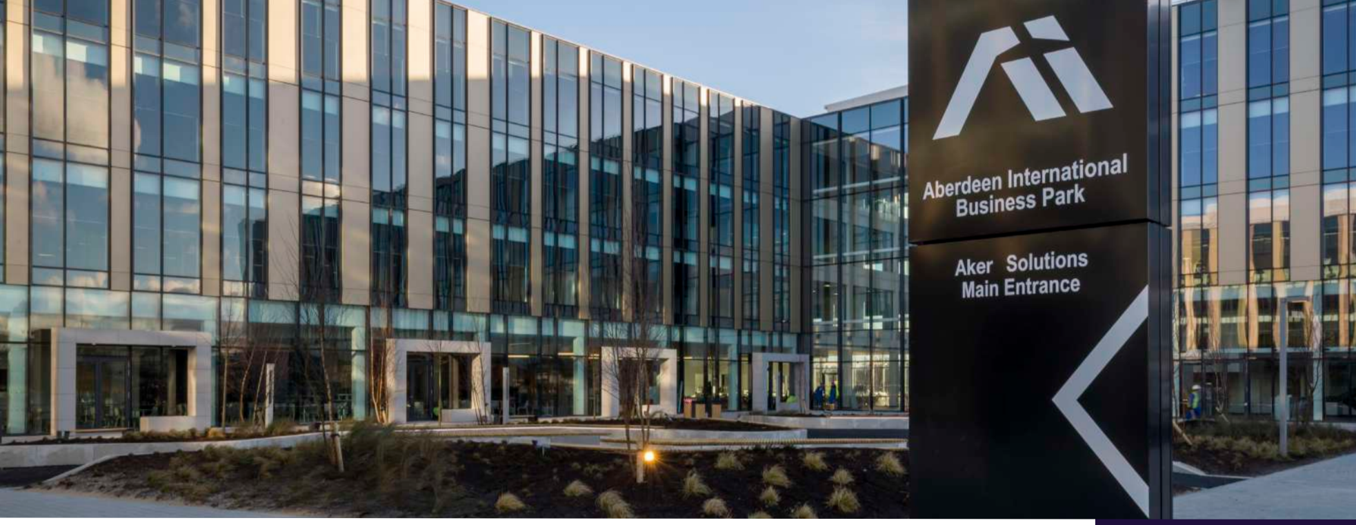
Aberdeen International Business Park (AIBP)
