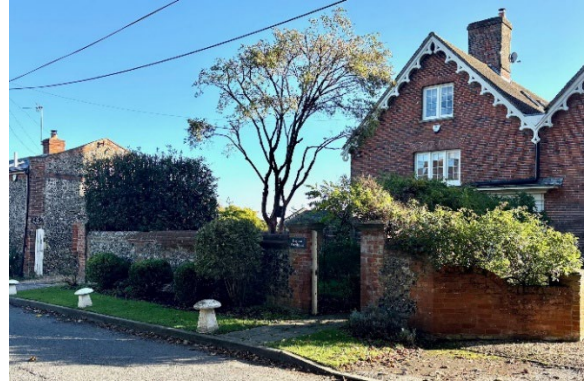
Image 11: Flint walls, Heydon Farmhouse, Fowlmere Road (looking south)
