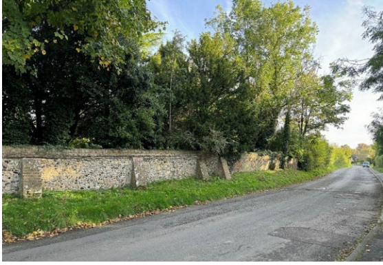
Image 10: Flint walls, Heydonbury Farmhouse, Fowlmere Road (looking towards the village core)
