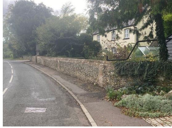
Image 17: Flint wall at Hill Farm, Chishill Road (looking away from the village core).
