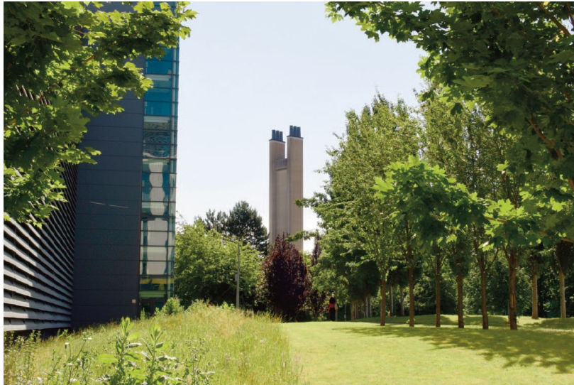
Image 65: Addenbrooke's Hospital incinerator chimney Image Credit: CBC Ltd
