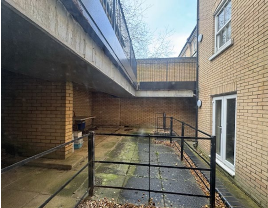
Image 17 - Position of lower ground floor windows within terrace (image shows 179 St Matthew's Gardens)
