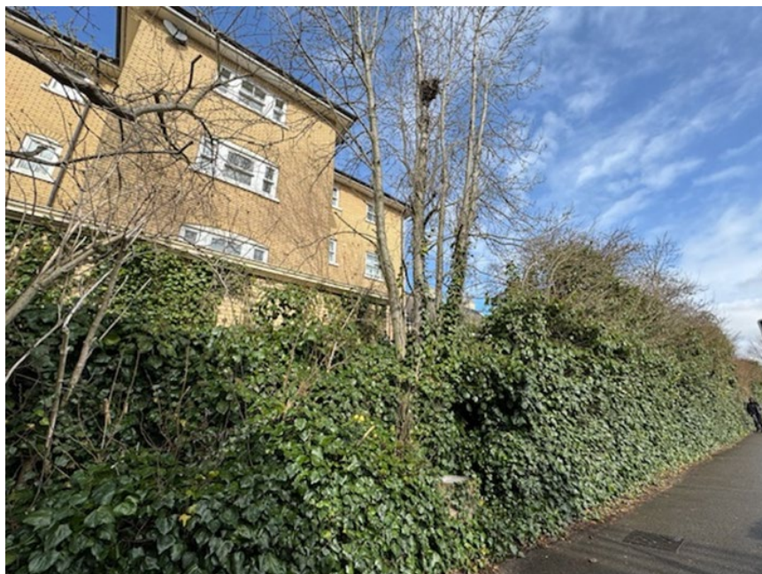
Image 10 - Application site boundary to St Matthew's Gardens (March 2025)
