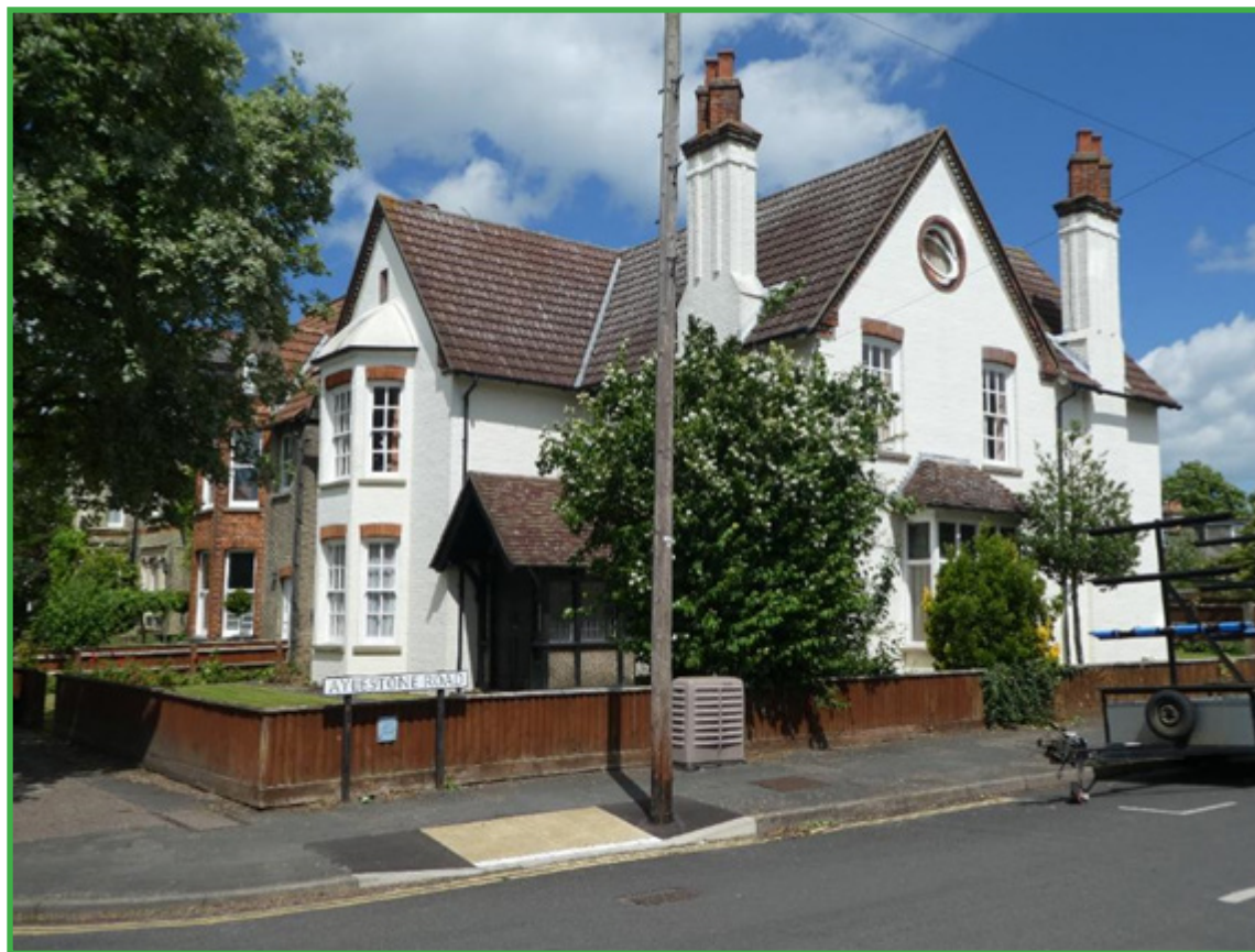
St George's House, De Freville Avenue
