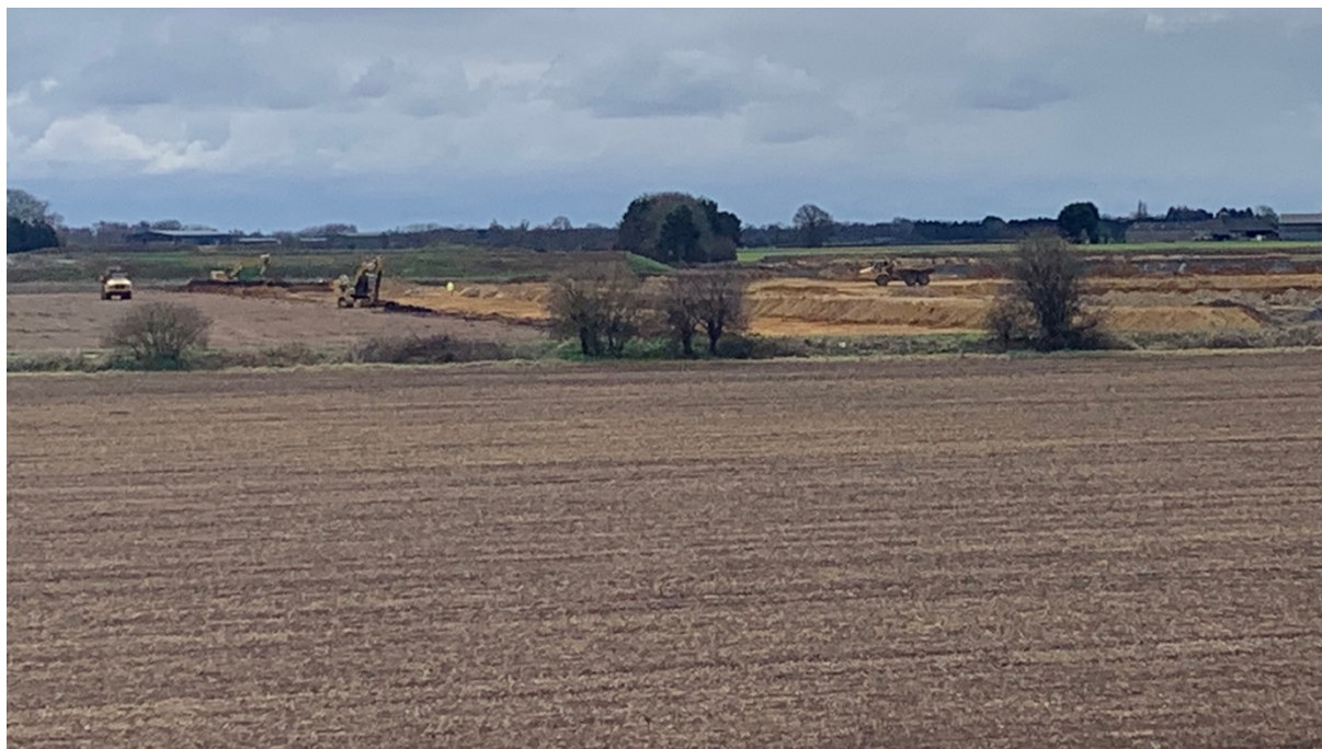
Top soil removal by 2 x excavators and 2 x ADTs on Phase 4. Looking south from The Site
