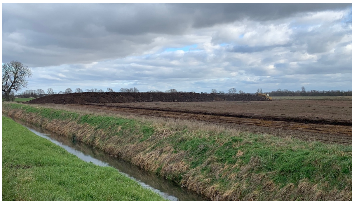
Top soil deposited at the eastern edge of Phase 5
