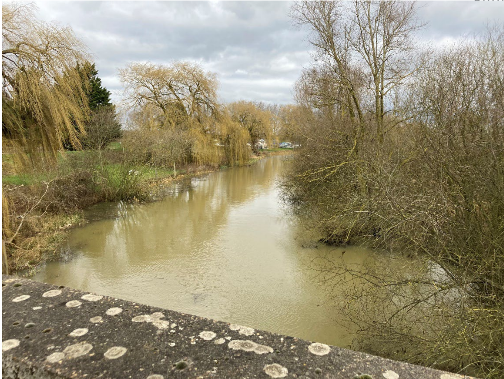
Figure 4 View east along the river corridor from Twenty Pence Bridge
