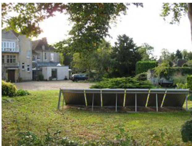
Example of freestanding solar panels installed in the garden of a Listed Building
