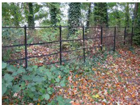
Example of park or estate railings
