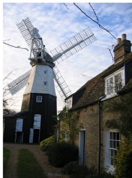
Impington Smock Mill
