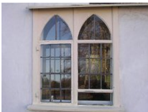
Example of leaded light windows (one on left also has secondary glazing)
