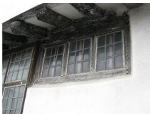
Example of leaded light windows (one on left also has secondary glazing)
