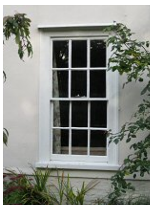
Example of a sash window
