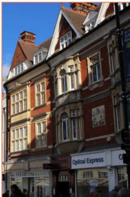
Detailing to No. 1 Market Hill
