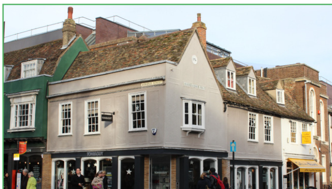
Timber framed buildings
