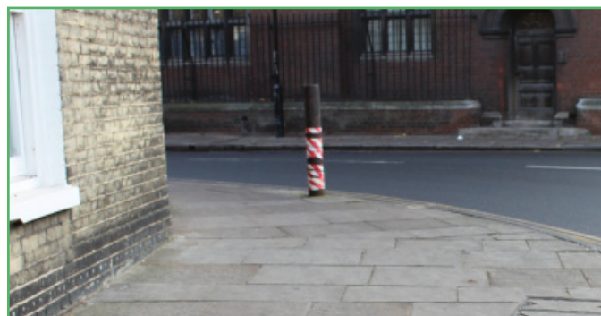
Poor paving and bollard by No. 1 Emmanuel Street
