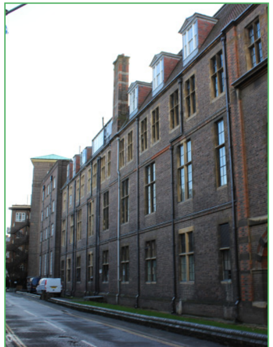
The Sedgwick and laboratory buildings to west side
