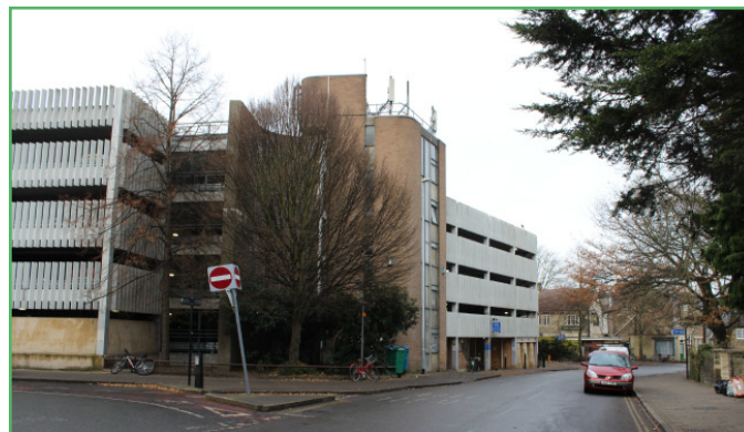
Multi-storey car park
