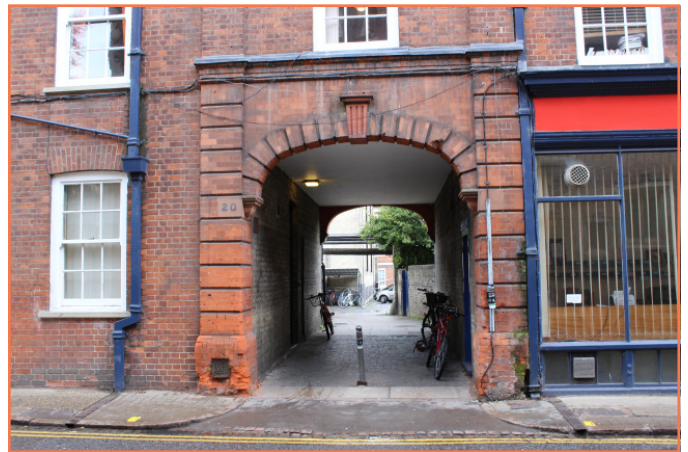
Wooden block paved tunnel
