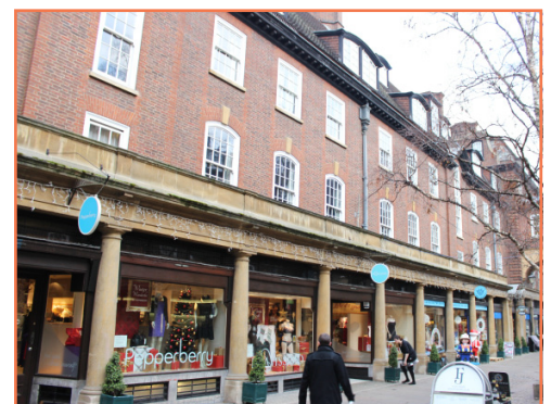
Shopfronts and dormer windows
