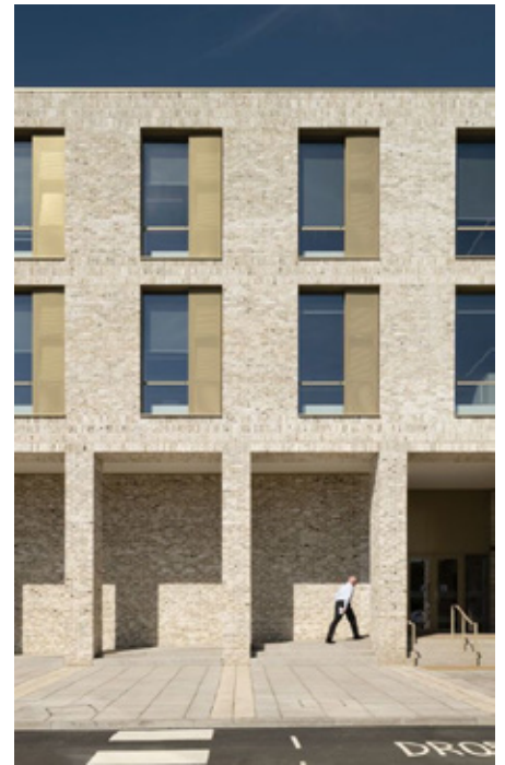
Predominantly buff/gault brick with complimentary reveal tones. Judge Business School, Cambridge, Stanton Williams
