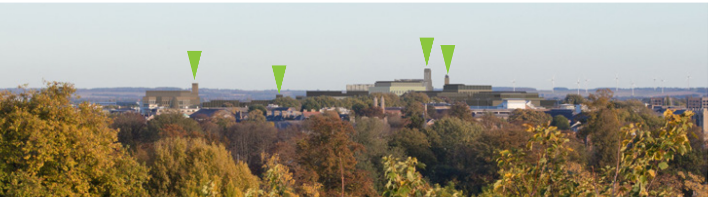
Flues evenly distributed, with the tallest flues grouped when viewed from Castle Hill Mound
