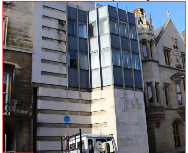
The building on the site of the Black Bull Inn
