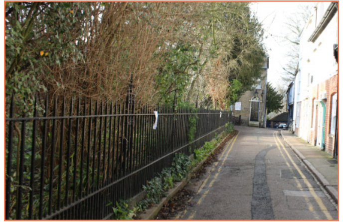
Little St Mary's Churchyard and railings
