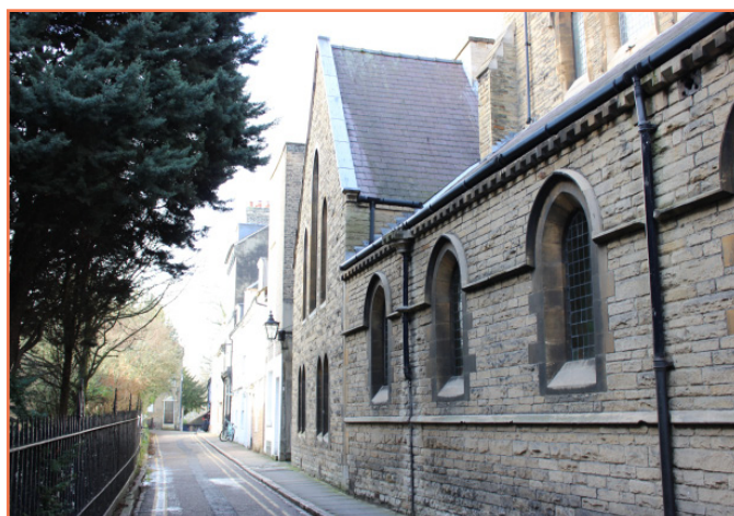
Side elevation of Emmanuel United Reformed Church
