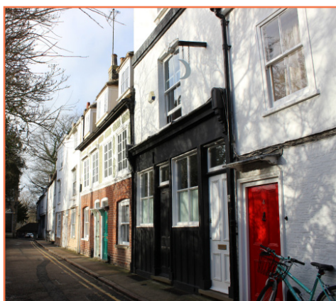
Two storey scale buildings with timber-framed sash windows
