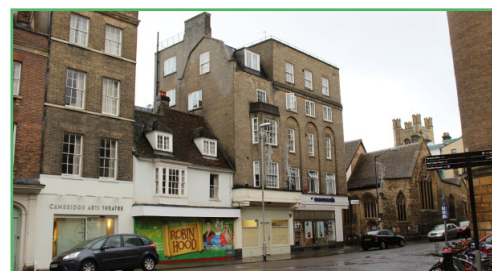
Buildings to the west
